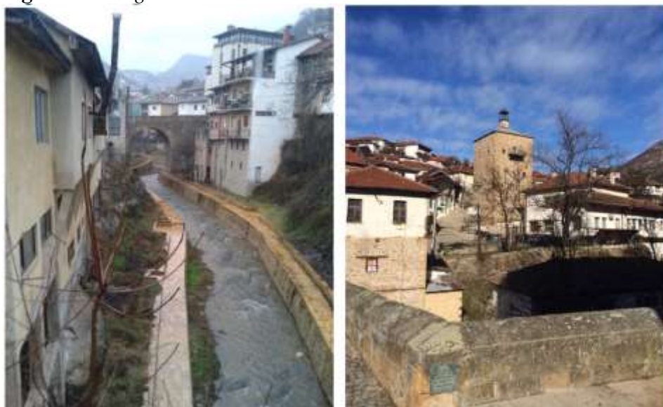
Figure 8: Bridges in Kratovo
